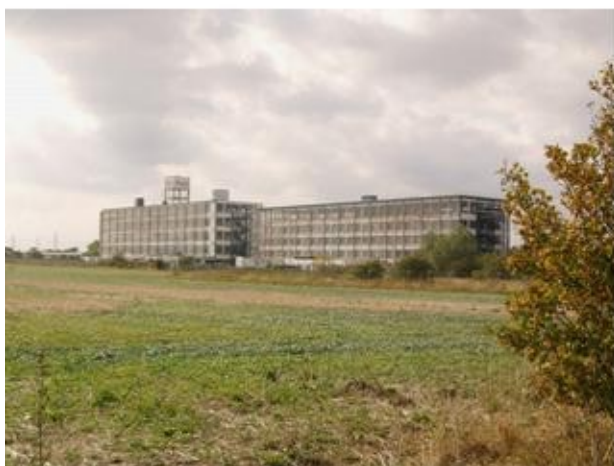
The British Bata Shoe Company's Factory, East Tilbury, Essex
